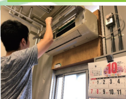
Air conditioner filter cleaning
